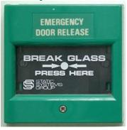
The security system installed within the buildings provides a controlled means of entry and exit. In a fire emergency the doors will 'fail-safe', i.e. unlock when the fire alarm sounds, and can be opened by pushing the door. If this hasn't worked, green emergency door release call points are located on the exit routes – press the panel and it will override the security systems
