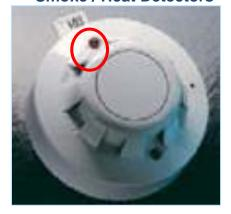
Located in all rooms of the building. If this device has activated the alarm, you will note that the small red LED of the side of the detector will either be on constant or flashing quickly.
