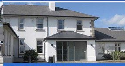
Rye, Winchelsea and District Memorial Hospital
